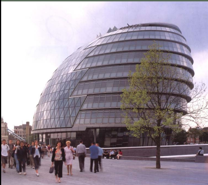
Foster & Partners: Greater London Authority (városháza), London, 2003
